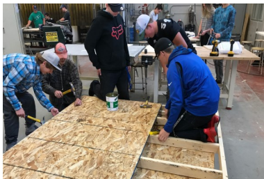
Construction class builds shed for community
